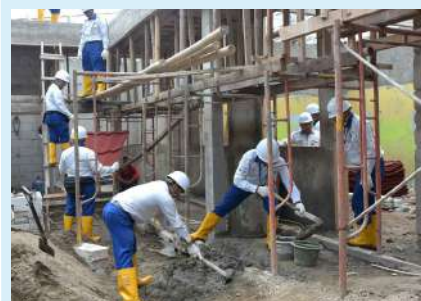
Kindergarten School Construction
